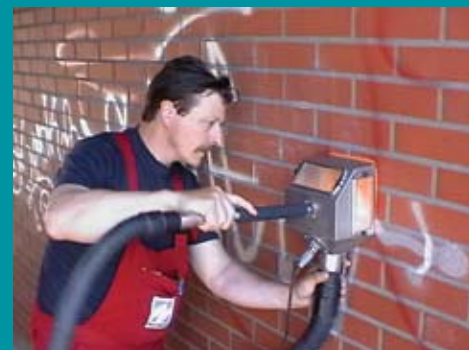
Background Surface Brickwork: Bricks and joints can be cleaned easily whether it be for removing graffiti, efflorescence or discoloring.
