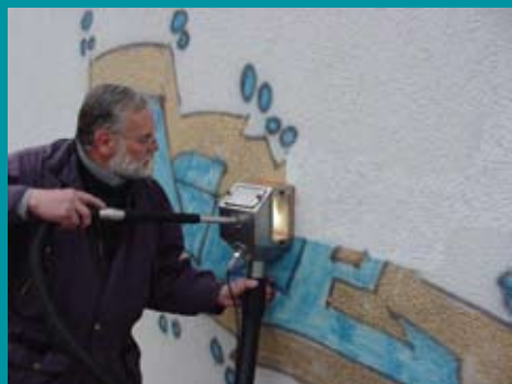
Background Surfaces, Plaster: Colored plaster, painted facades and especially thermal insulation system can be optically cleansed.
