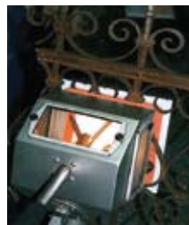
Derusting of metal items: Derusting of wrought – iron fences without unnecessary dismantling.
