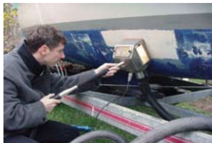
Precise removal on boathulls- Layers of paint on the underside of hulls can be removed by using hard granules. The jet can enables the exact edges of areas to be marked out without the use of masking tape. Optimal for use by smaller shipyards and clubs.
