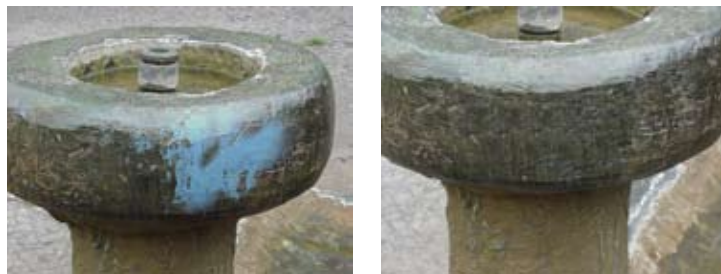
Careful removal of unwanted surface layer: By using nutshell granules graffiti was removed from an old bronze fountain without damaging the typical surface oxidation.
